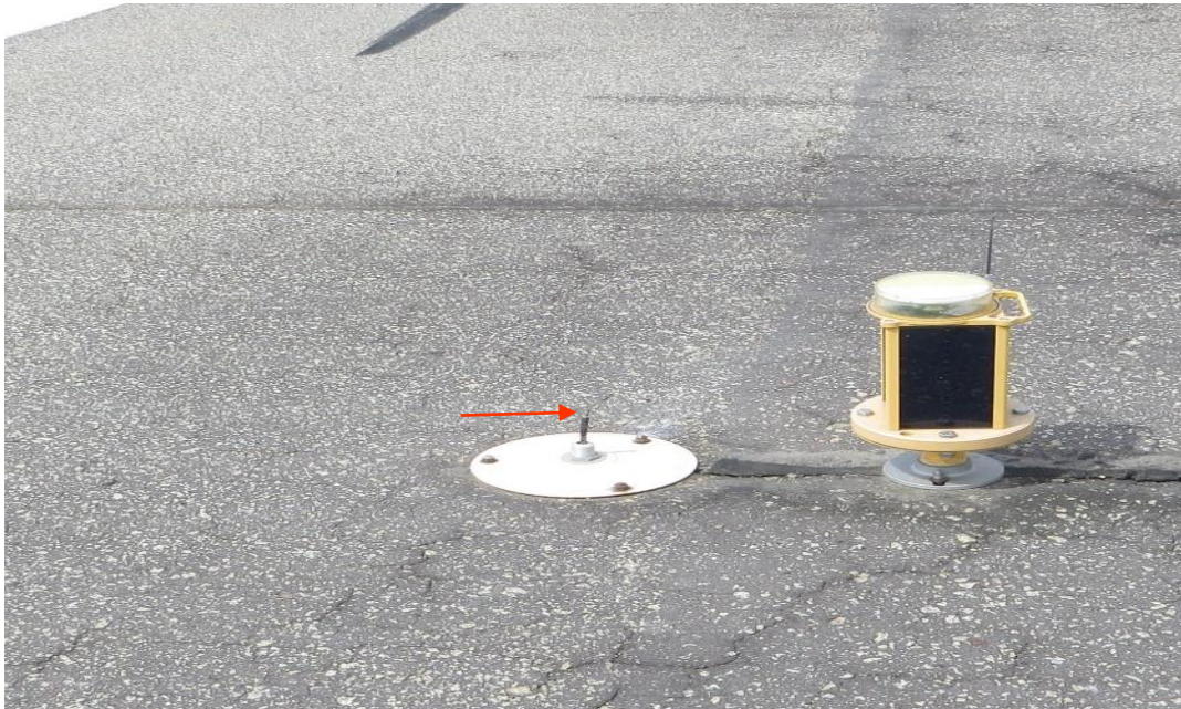
Figure 2: Damaged runway edge light
