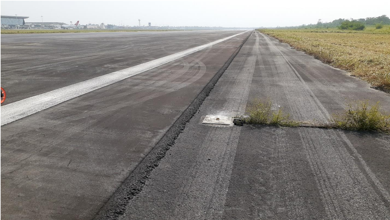
Figure 10: A photo of the tyre marks from the right main wheel tyres on the runway shoulder
