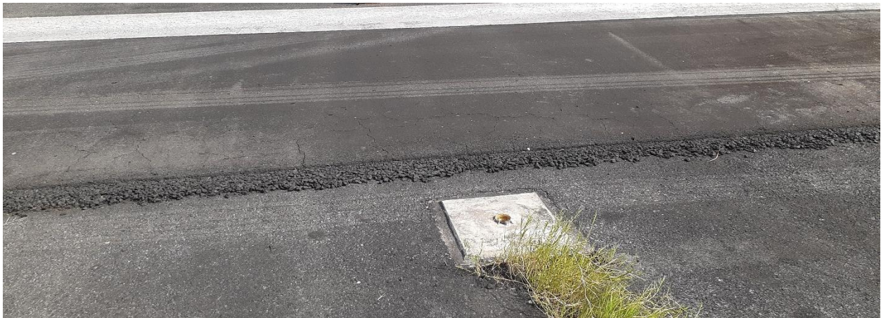
Figure 9: Photo of one of the damaged runway edge lights
