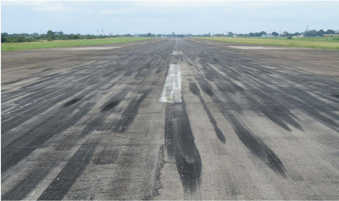
Figure 2: Rubberized touchdown zone of runway 05
