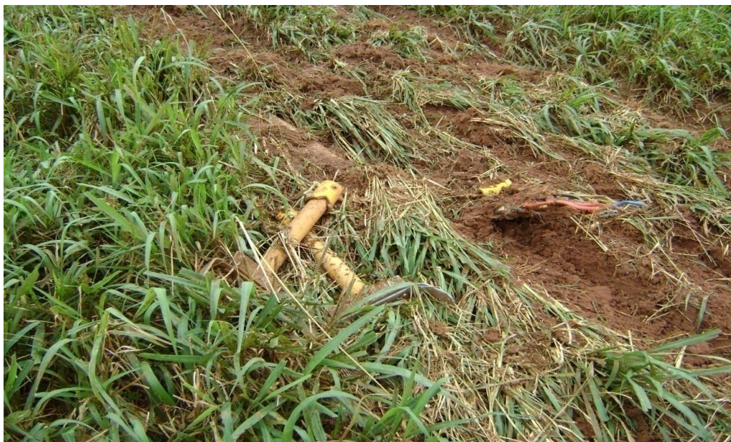
Figure 10: Damage to the approach lights of runway 23
