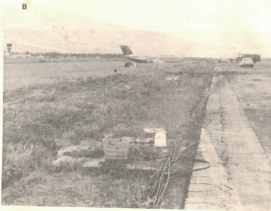
Photograph showing the type of hazardous refilling job performed along the runway shoulder.
