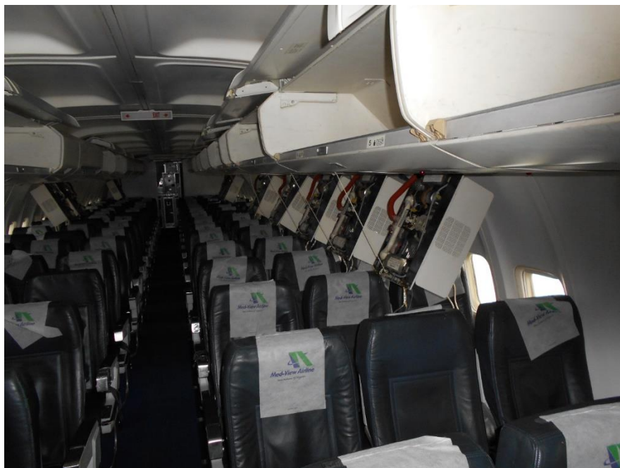
Figure 3: Photo of the passenger service units (PSUs) in open position when investigators arrived
