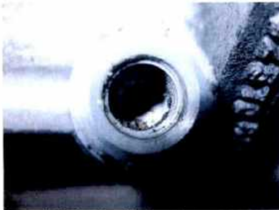
Figure AI-21: Overboard drain port
