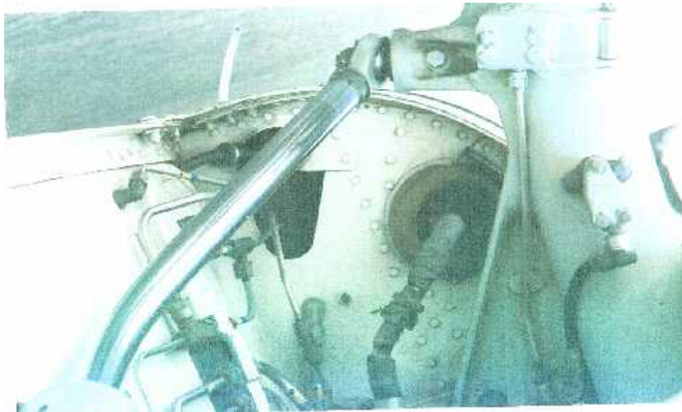
Fig. 1.12c Photograph showing bent strut
