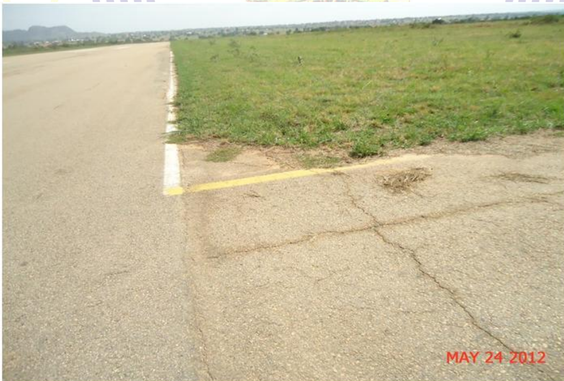
Figure 2: The Unclear exit 3 Markings
